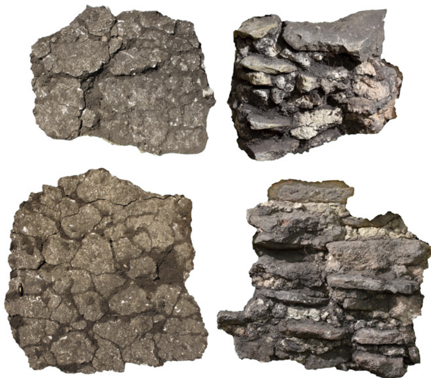
FIGURE 1.4 Pohansko near Břeclav – north-east suburb. Church No. 2. Two blocks of the collapsed walls of the apse recovered in situ, dimensions 30 × 43 cm and 48 × 46 cm.
